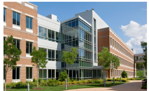
55 Network Drive, home to Exa Corporation
