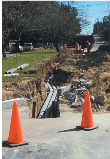
Norblom began work on this extensive utility project in 2000.
