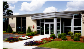
21-23 Third Avenue, home to Acronis, Inc.
